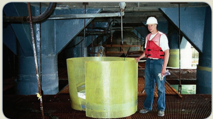
Fort Mason - pile strengthening
