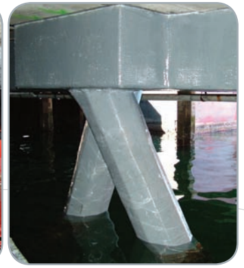
NASSCO Pier, California - corroded piles repaired
