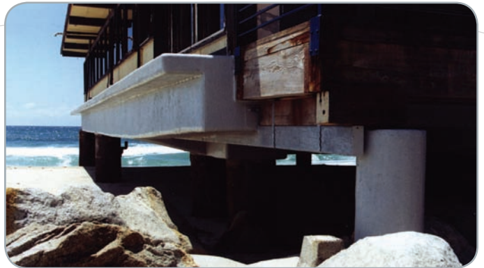
Redondo Beach Restaurant - beam, pile & slab repairs
