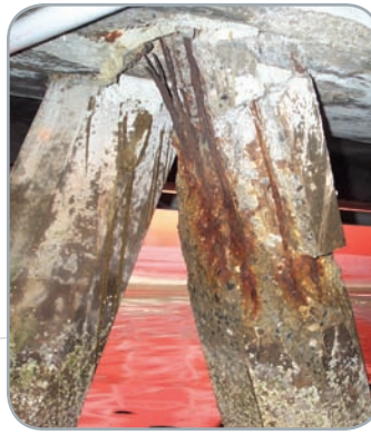
NASSCO Pier, California - corroded piles repaired
