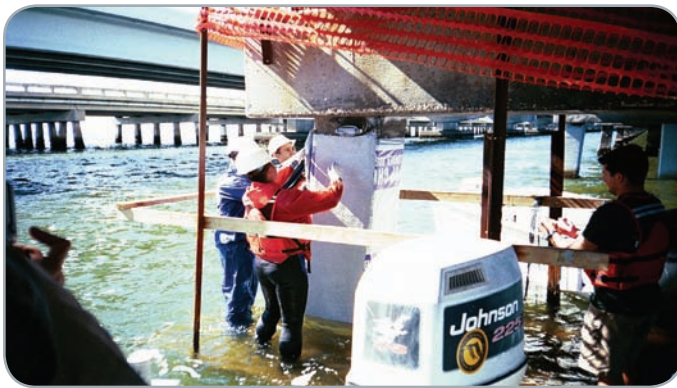
Friendship Trail Bridge, Florida - corrosion mitigation
