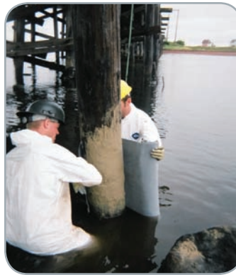
Darnley Bridge, Canada - wood pile retrofit
