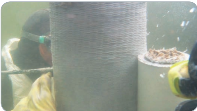
Canada East - wood pile repairs
