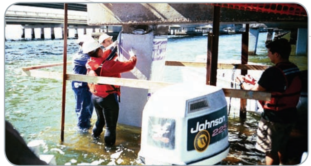
Friendship Trail Bridge, Florida - corrosion mitigation
