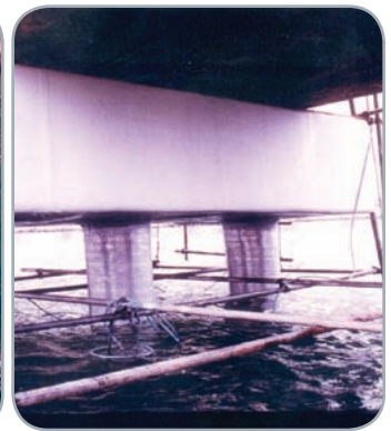
SK Port - beam, pile repairs
