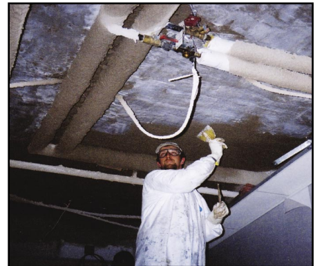
Tyfo® EI-R being applied around obstacles
