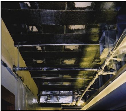
Tyfo® Carbon Composite applied
