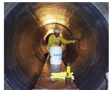
Specialty scaffolding is designed to span the spool length to allow access to the entire pipe face
