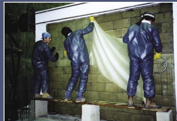
Seismic strengthening of masonry-infilled frames using the Tyfo® SEH System
