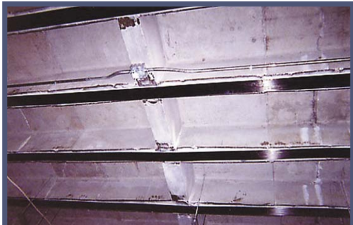
Tyfo® UC Carbon Laminates were used to strengthen these library floor joints
