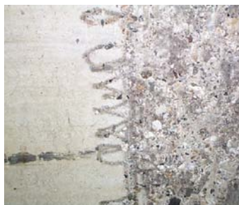
Surface preparation with hydro blasting to achieve the required 1/16" minimum amplitude
